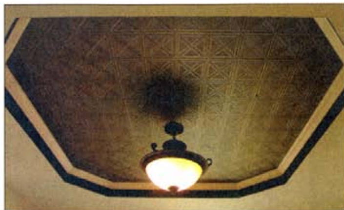
Tray ceilings inside 640 Stuart St. received special treatment with patterned and painted panels.
